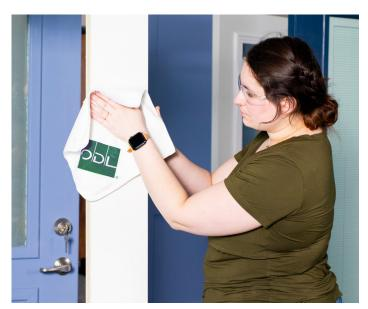
**STEP 4:** Clean both sides of door by wiping with rag. Ensure door is free of dirt, dust and debris. Isopropyl alcohol may be used to wipe down door to ensure a clean bonding surface.
