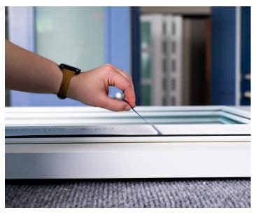
**STEP 6:** Remove release liner from tape on inner frame.
