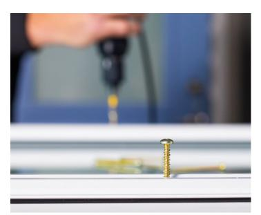
**STEP 8:** Drive all screws starting with the 2 center screw locations using the provided installation torque of 17.7 inch-pounds. **Do not over tighten screws.**
