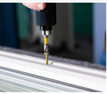
**STEP 2:** Remove shipping screws from inner frame and set aside.
