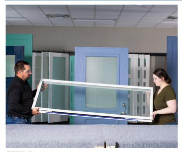
**STEP 1:** Inspect frame and set on a flat surface with exterior side down.
