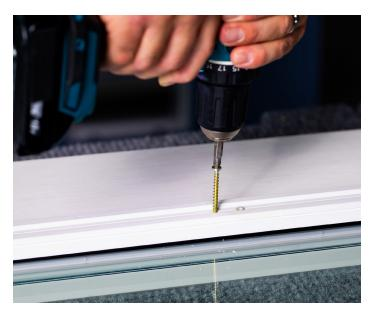
**STEP 2:** Drive screw using the provided installation torque of 17.7 inch-pounds.
