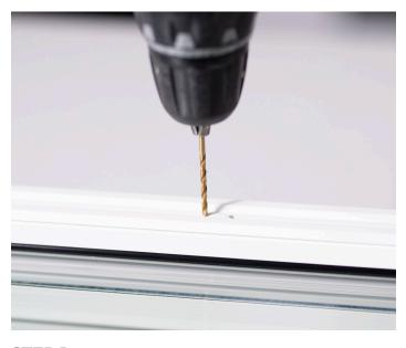
**STEP 1:** Line up new location a half inch from original. Drill a new hole through the inner frame using an 11/64" drill bit. **Do not go into the outer frame.**
