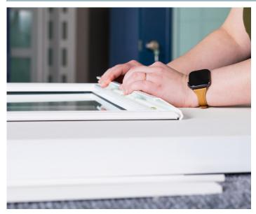
**STEP 1:** Start with short side cover along top of the frame. Center cover along frame. Starting with outside edge of cover, hook and rotate while snapping into place along glass side.
