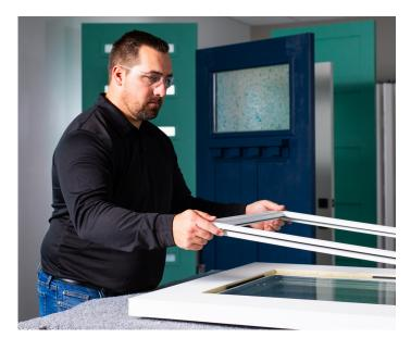
**STEP 7:** Assemble inner frame into alignment H-Channels, ensuring it is properly seated on all sides.
